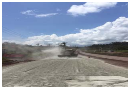
Pengupasan tanah eksisting Sta 8+00 – 8+220
